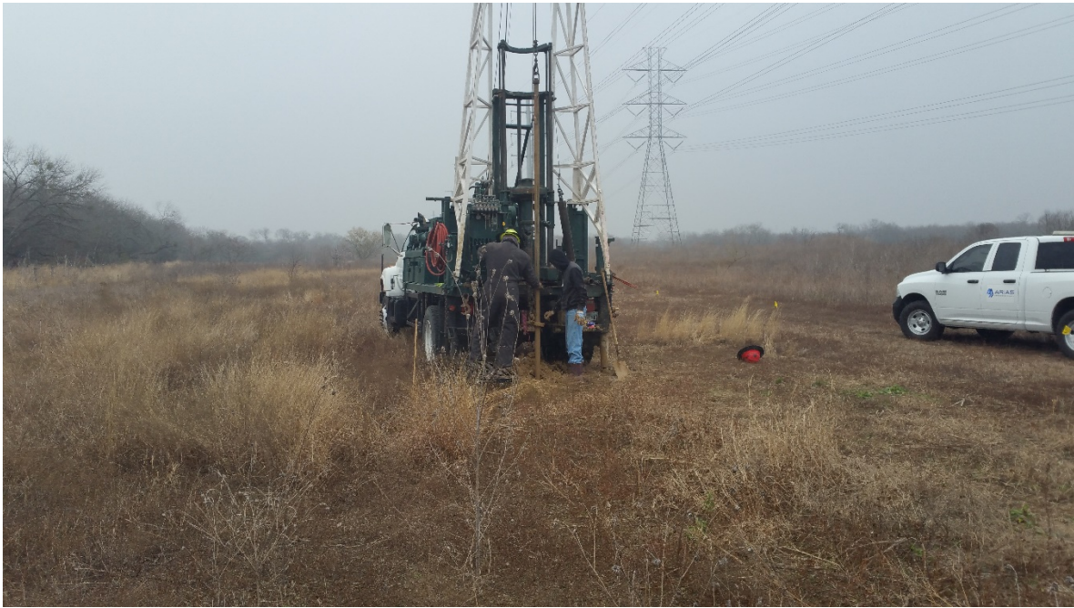
Photo 1 – View looking at Boring 103 drilling operations.
